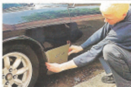
Decent repair sections are now available for all common rot spots at £30 a throw.
